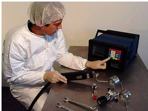
Fig. 6 preparation for orbital weld of gas pipes
