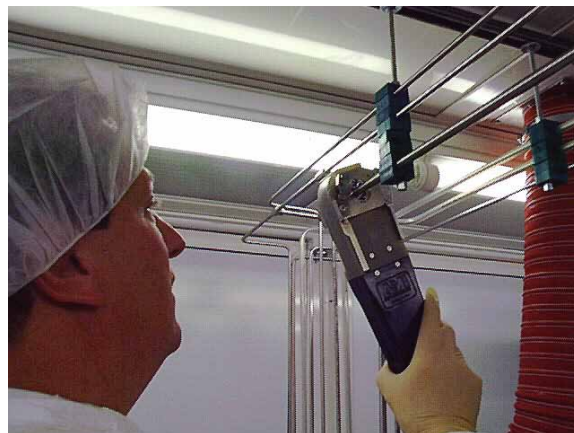
Fig. 7 orbital weld of gas pipes
